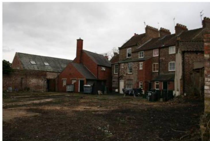
FRONT AND REAR VIEWS OF EXISTING THREE STOREY RETAIL UNITS TO THE SOUTHERN BOUNDARY
